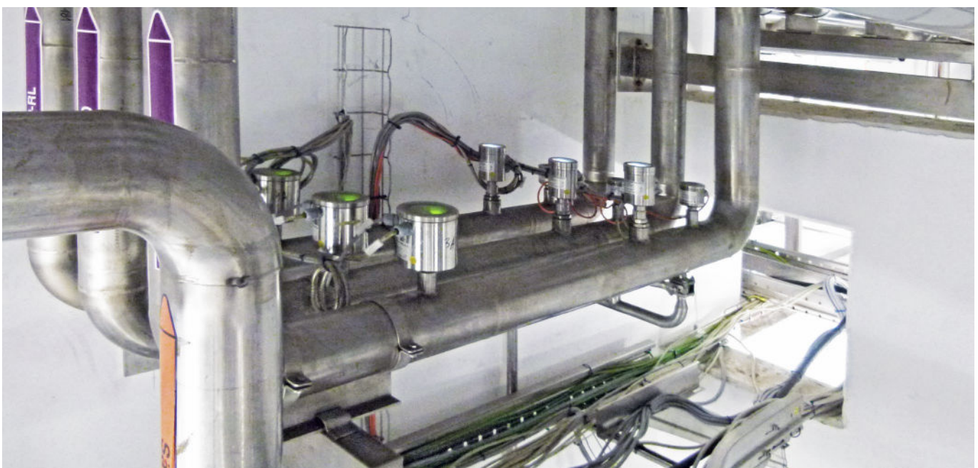
ITM-3, ILM-4 and FWS sensors for the precise phase separation
