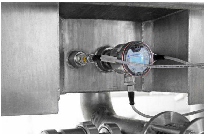
Common practice for storage and maturation tanks: Simple installation of hydrostatic level sensor (here L3 Neo), temperature sensor and point level switch on the underside of the tank
